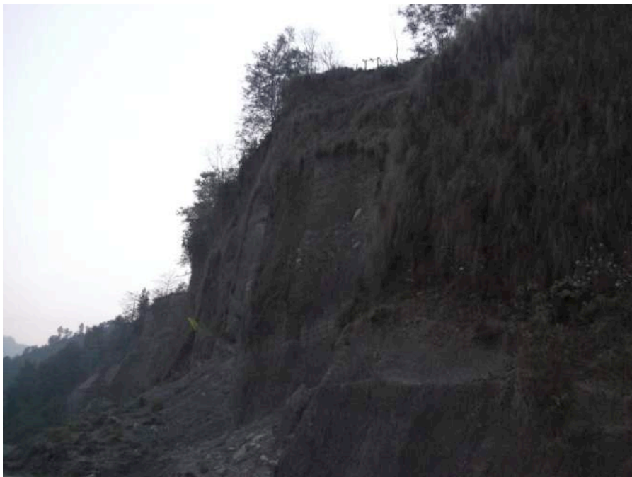
Erosion in Wantang Khola, tributary of Seti river
