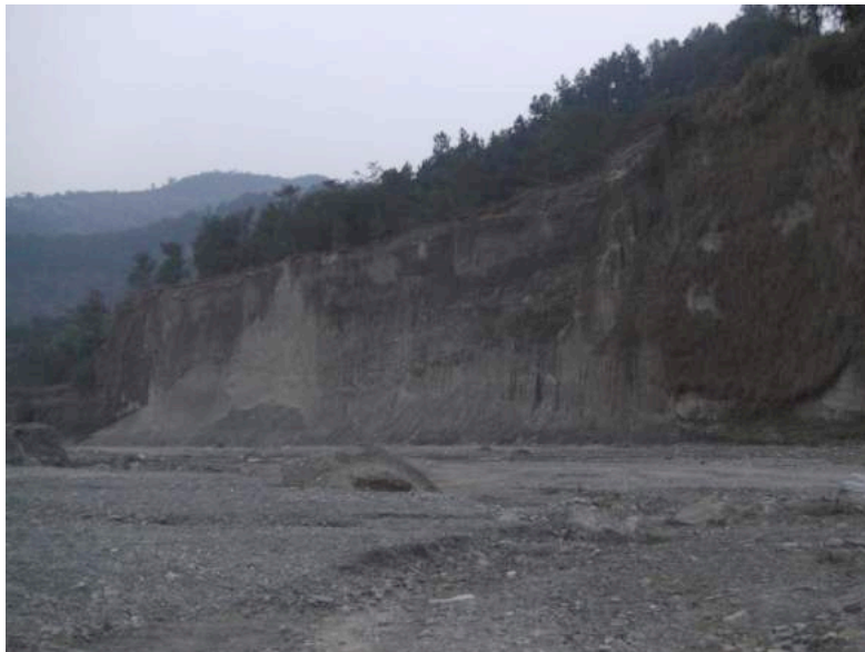
Erosion and landslides in Basin (Source: DP Upadhyay, January, 2014))
