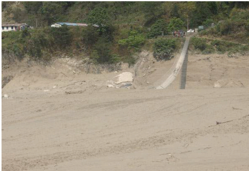
Suspension bridge after Seti flood in 5 May 2012, Photo credit: Kantipur daily
